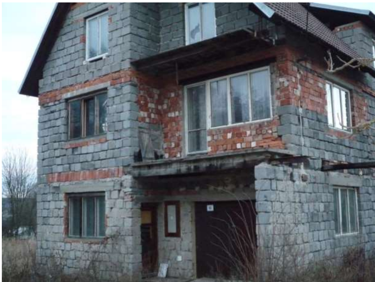
Fig. 3: Unsuitable combination of perimeter wall materials (Hlavsa P., 2012)
