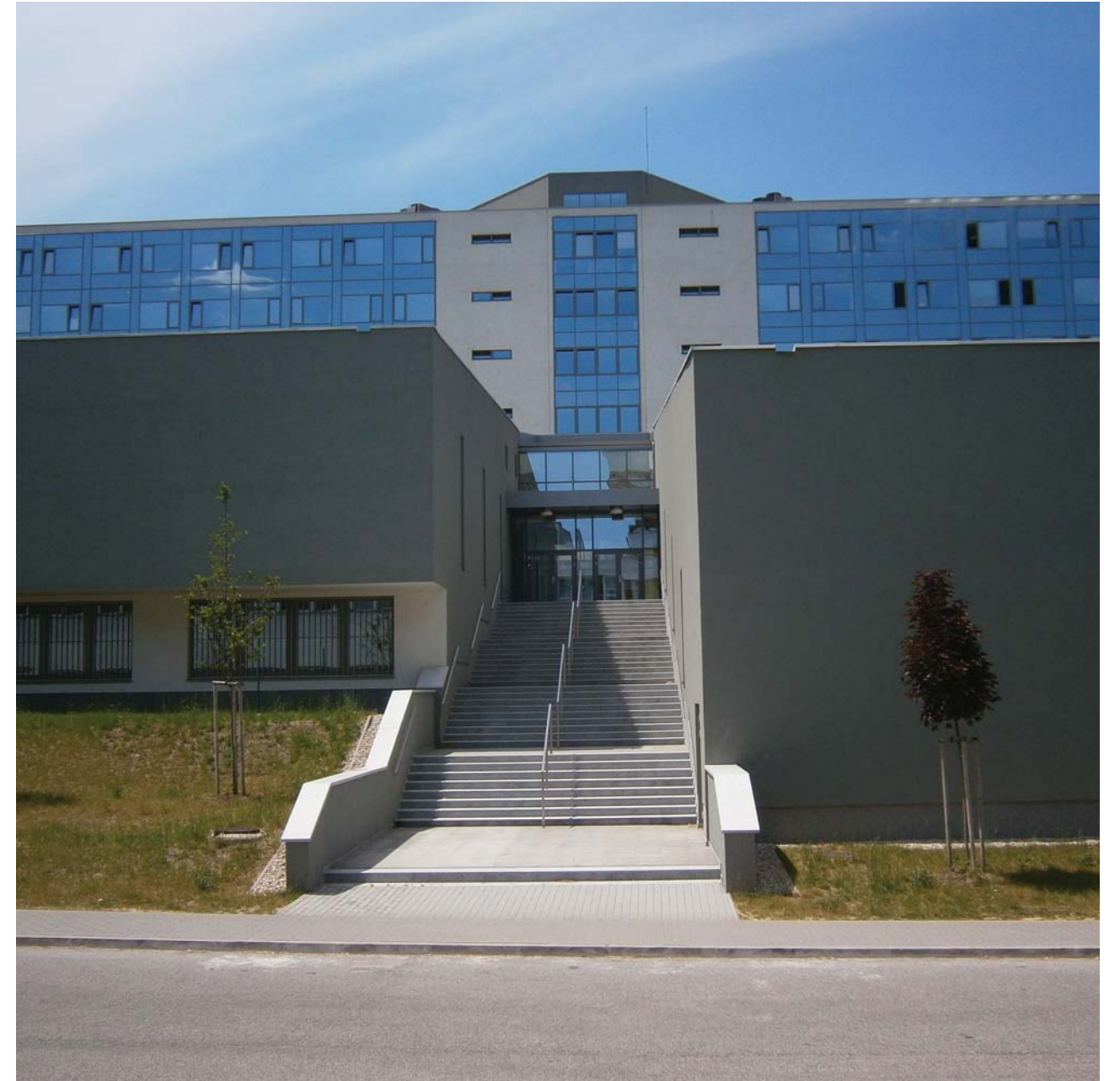
New building of the Faculty of informatics and information technologies
