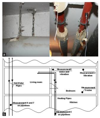
Figure 4: Source of vibration and enclosed spaces (a) suspension of hot-water (in left old) and heating pipes (in right new) and (b) floor plan of the flat
